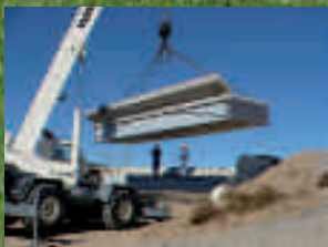
Composite Railroad Bridge Passes Live Load Test with Advantex® Reinforcements
