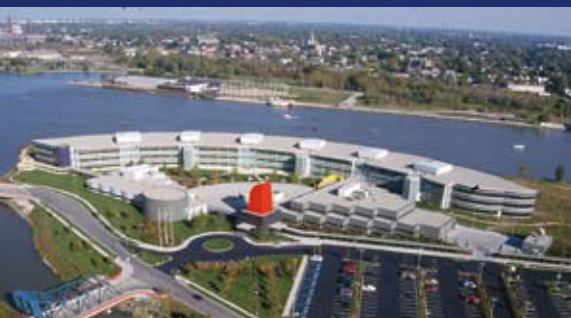
Energy and environmental footprint reduction projects impact all Owens Corning facilities.
